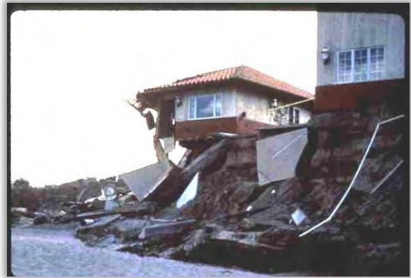
Figure 1-20. Erosion can destroy a building that is above the flood level.
