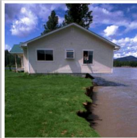
Figure 1-5. Riverine erosion can undercut structures
