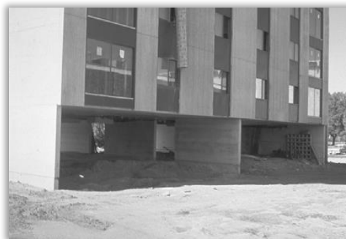
Figure 12-2. Building elevated on parallel stem walls.
