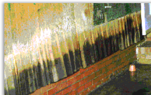
Figure 1-19. Prolonged exposure to water and “wicking” can destroy wood and gypsum walls.
