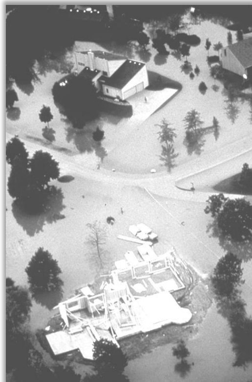
Figure 12-1. These two new buildings elevated on fill plus freeboard were not damaged by this 100-year flood.
