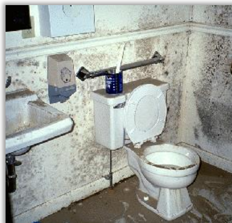
Figure 1-14. Mold and mildew can grow quickly after a flood
