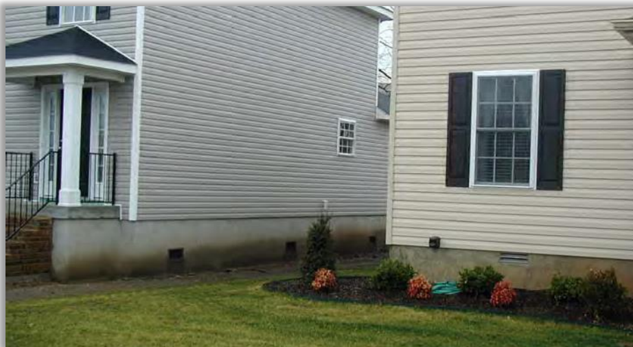
Figure 12-6. The house on the left has compliant crawlspace openings. the openings in the foundation on the right are too high.
