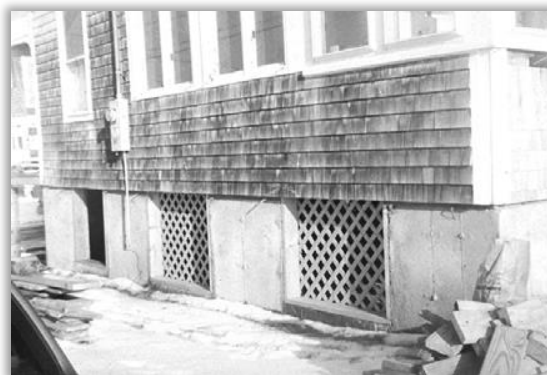
Figure 12-3. Building elevated on crawlspace with openings.
