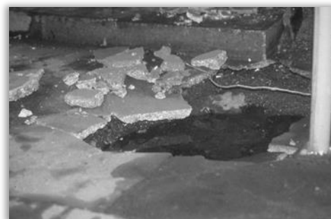
Figure 3. This basement floor broke from hydrostatic pressure.
